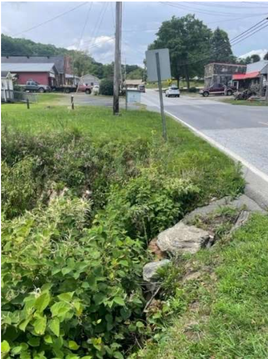
Figure 2-5: Culvert at East Main Street and Meadow Road, Looking West
